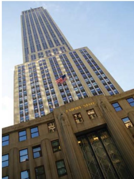
The Empire State Building: A sustainable retrofit has yielded huge savings on energy costs
