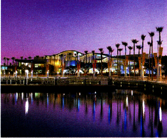
The 88,000-square-foot Aquarium of the Pacific in Long Beach underwent an energy audit, after which time engineering drawings and specifications were prepared to replace boilers and installing controls.
